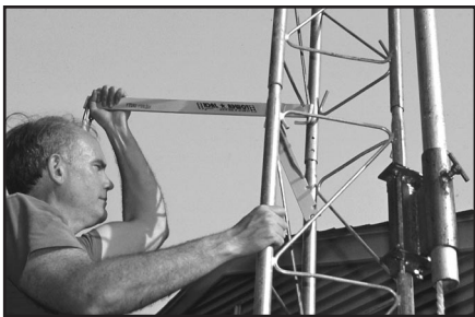
Figure 2—The Tower Jack provides the leverage needed to easily separate stubborn sections.
